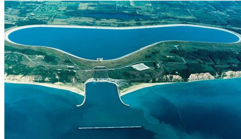
Hydro Pumped Storage
