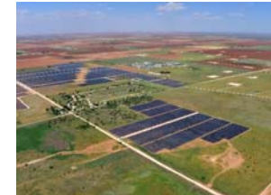
102 MW Lamesa Solar
